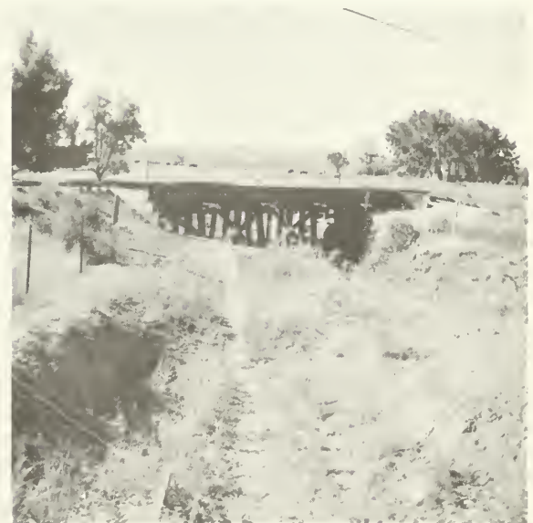
Looking southeasterly from SOUTHEAST ENTRANCE, showing trail under rail- road bridge
